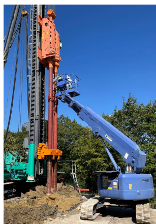
写真-4 孔曲がり計測状況 Fig-4 Borehole Deviation Measurement in Progress
